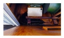
We could not see blades as fan was running during survey; however fan blades seem to be in a fair to good condition. The fan housing however has puddles of grease forming below motor. The walls of the housing have high levels of contamination as the WFTT results show.
