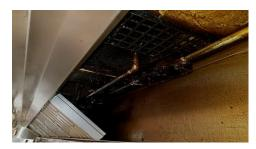
Grills are full of grease and carbon contamination, will have to remove to clean riser above and grills.
