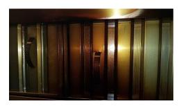
All the Baffles had high levels of contamination, the worst of the Baffles were above smoker, grease and carbon deposits were baked onto Baffles and suggest regular cleaning by KPs. These need to be first coated in Sodium Hydroxide, once the chemical has had an effect clean with pressure washer in conjunction with Ubik.
