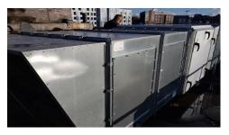
There is a total of approximately 10 metres of ductwork on the roof, the walls, ceiling and floor of ductwork has medium to high levels of contamination.
