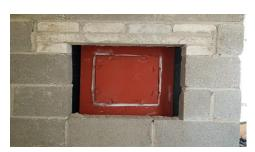
Access to riser is on each floor of building, there is a total of 5 access panels that are fitted in fire rated ductwork. The access doors are in a poor condition and had trouble to open doors; however we have spare doors and will fit should any damage occur.
