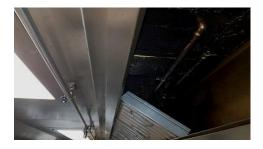
Canopy has extremely high levels of both grease and carbon deposits; this will again be coated in Sodium Hydroxide, scraped then coated again. The contamination is baked on and will be extremely hard to remove and may have to be done over two nights to achieve the standards we required.
