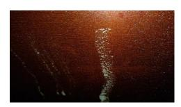
Grease contamination to hard for conventional WFTT, there are 4 risers that will need to be coated in Sodium Hydroxide over night, we must try and get riser back to bear metal.
