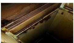
There is approximately 30 metres of riser from roof to header, there was medium to high levels of contamination as per WFTT. We will clean full riser, first by coating with Sodium Hydroxide then using a pressure washer in conjunction with Ubik degreaser. Because of the height of riser this may take two or more shifts depending on how chemical works.
