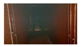
The Header is in a very poor condition with high levels of baked on grease contamination, this will have to be coated and left over night so that we can clean next day using a pressure washer in conjunction Ubik degreaser.
